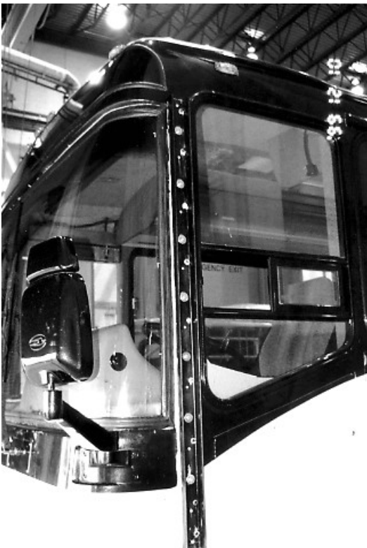
STEEL C-CHANNEL INSTALLED ON EXTERIOR OF WINDSHIELD PILLARS TO STIFFEN WINDSHIELD FRAME. MANUFACTURER DIRECTED MODIFICATION (914 TEST MILES)
