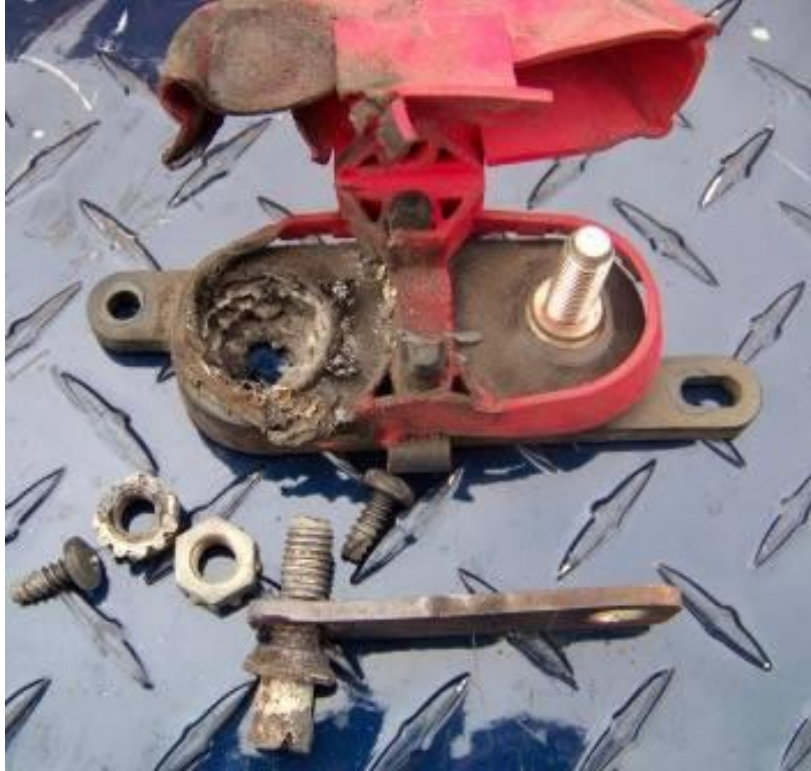
BURNT ELECTRICAL BUS BAR (14,526 TEST MILES)
