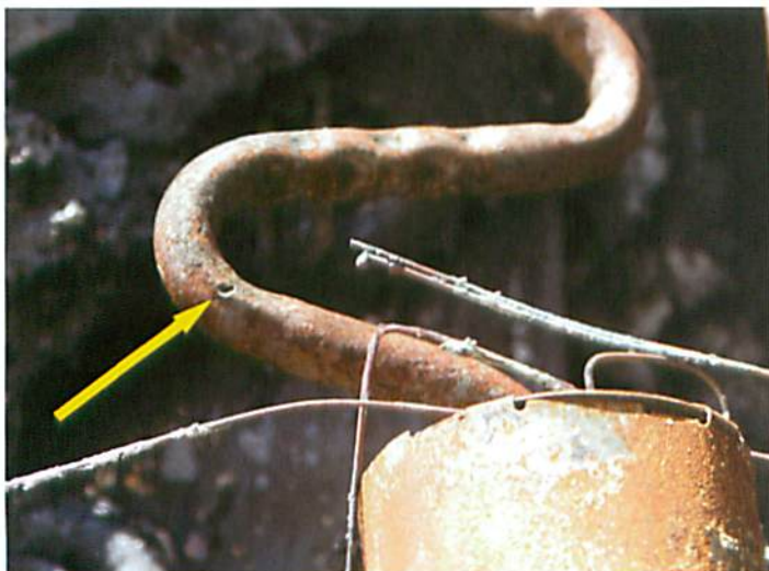
FIGURE 4—This unit exhibited evidence of electrical discharge damage. The area of electrical activity was consistent with the area of fire origin in this particular fire.
