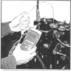
Testing the temperature at the discharge fitting.
