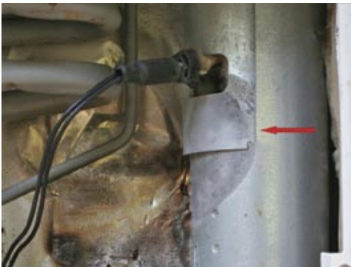
FIGURE 4 —Note the discoloration and radial heat pattern of the zinc coating on the steel sheet metal.
