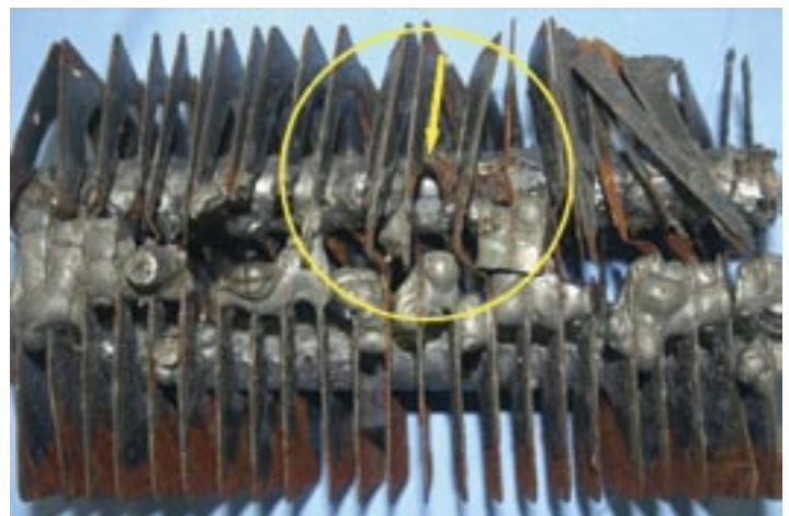
FIGURE 6 —Leak site created in a cooling unit condenser due to dissolution of the steel tubing wall in molten aluminum.
